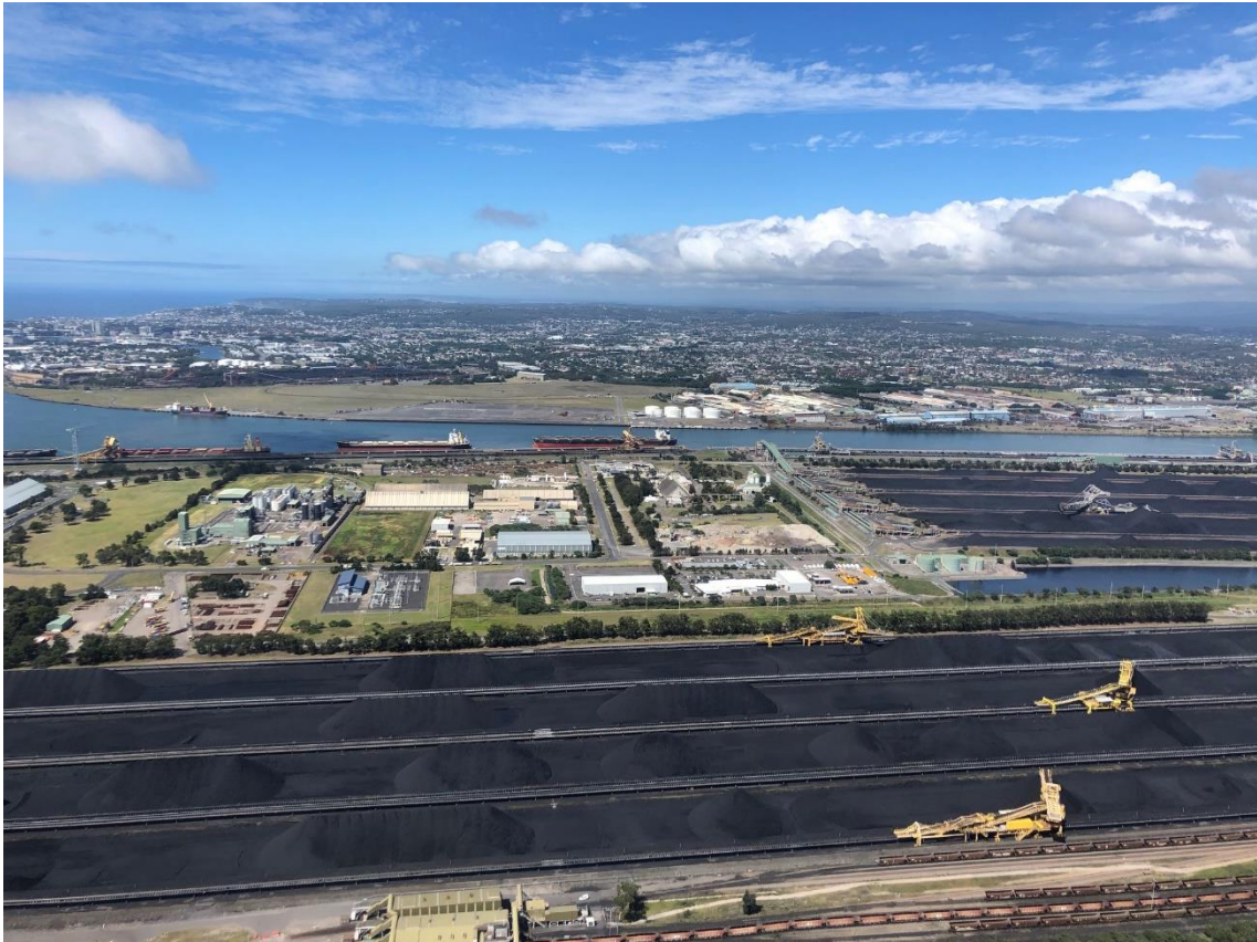
Coal shipping facilities at Newcastle Harbour (31 January 2022)
